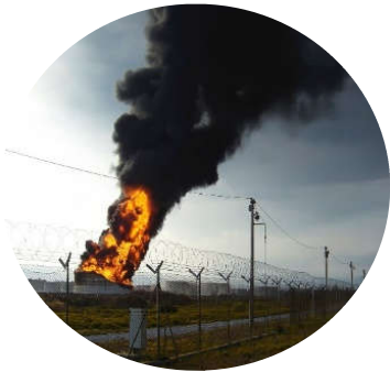
Failure of Industrial Systems
